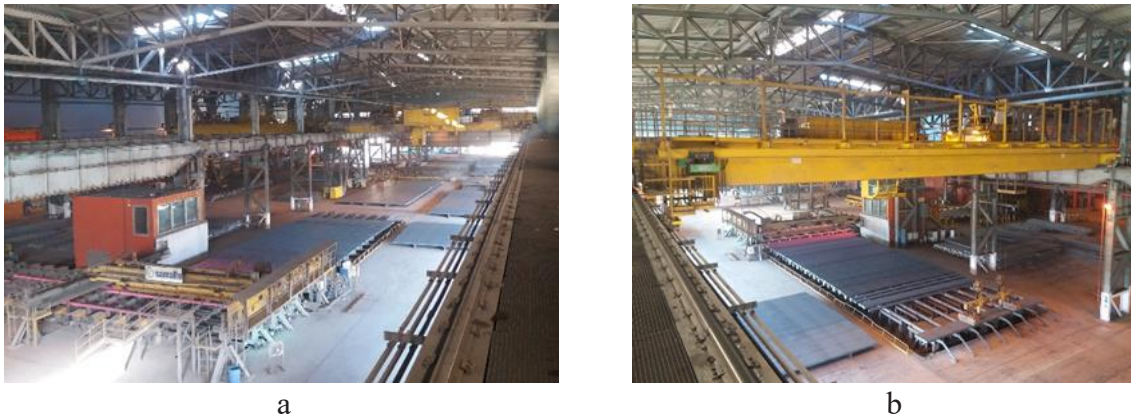
Fig. 1. The billet transport span in the SKS company a) South view b) North view.
