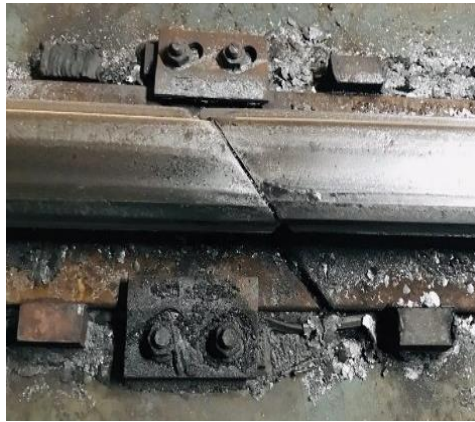
Fig. 11. A sample of the rail gap attachment which is designed and installed in the crane rail of the SKS Company.
