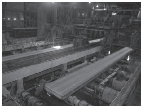
Fig. 1. Continuous casting unit in Mobarakeh Steel Company.
