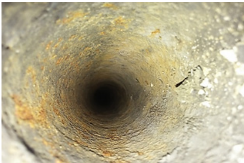
Fig. 5. The main burner nozzle in Bey No. 6.
