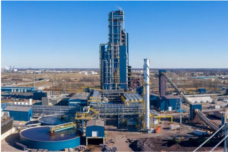
Fig. 6. A view of the new DRI production unit of the American Cliffs company [7].
