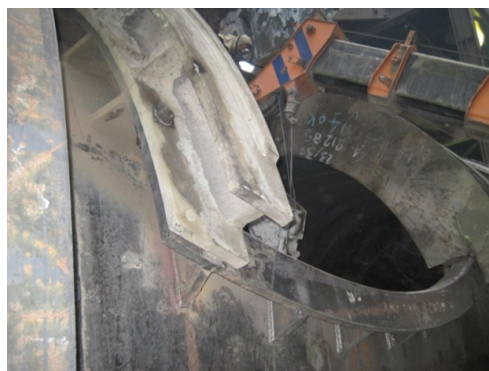
Fig. 1. The openings of Sarcheshmeh Copper Converter.
