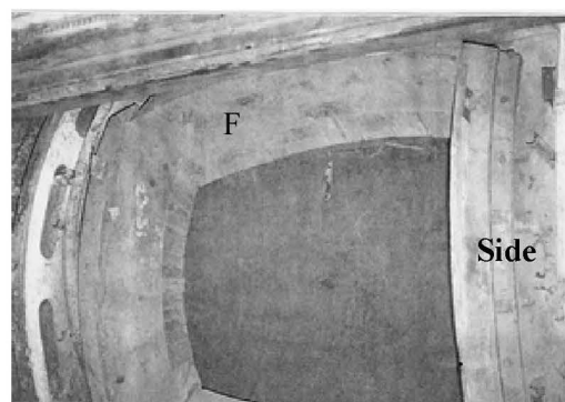
Fig. 1. The openings of Sarcheshmeh Copper Converter.
